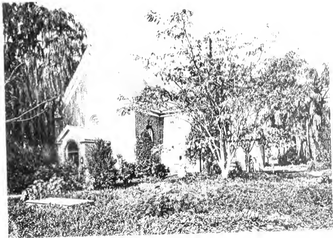
ST. JOHN'S EPISCOPAL CHURCH, HAMPTON, VA., NEAR OLD POINT.
